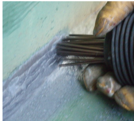
Fig 12 Needle gun cleaning
