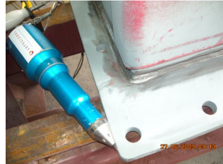
Fig 18 Treated weld surface
